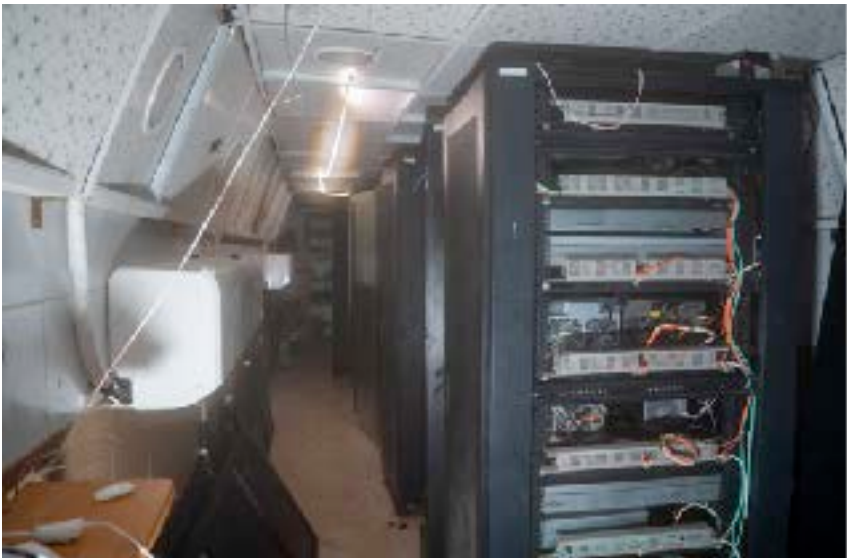
IDF revealed an underground HAMAS data center, directly beneath UNRWA headquarters in Gaza, used for intelligence and communications.
