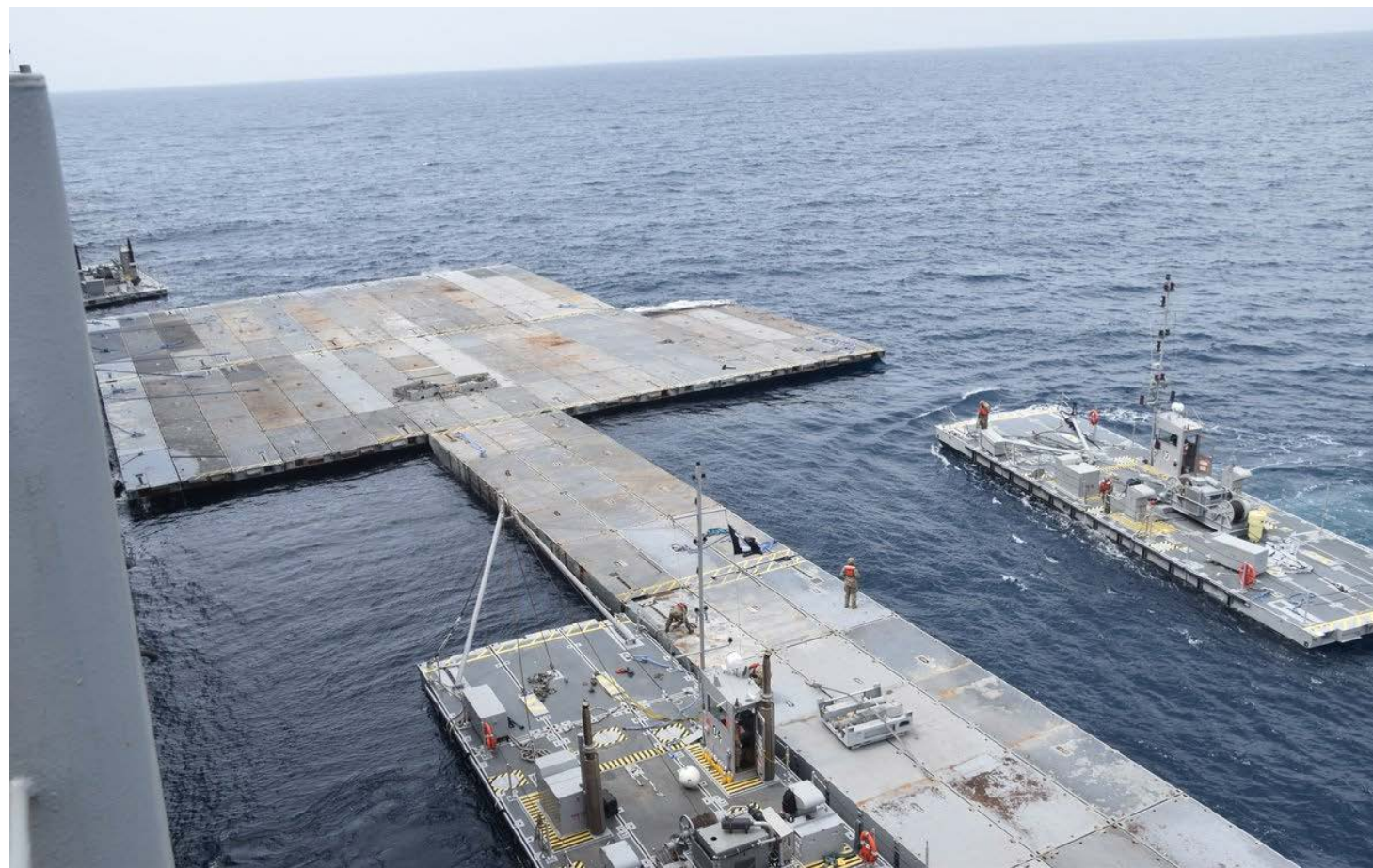
Image of US pier construction released by CENTCOM April 29 2024
